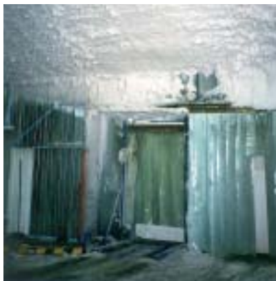
Icing-up leads to dangerous situations.
