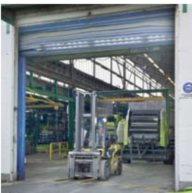
During loading and unloading the door remains open, without the indoor climate being disturbed.
