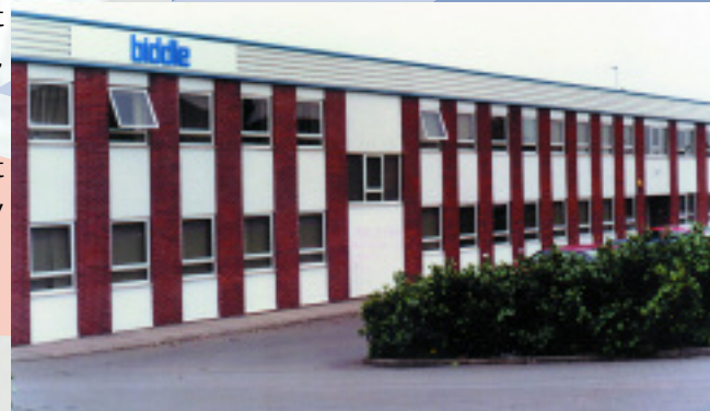
St. Mary's Road, Nuneaton
